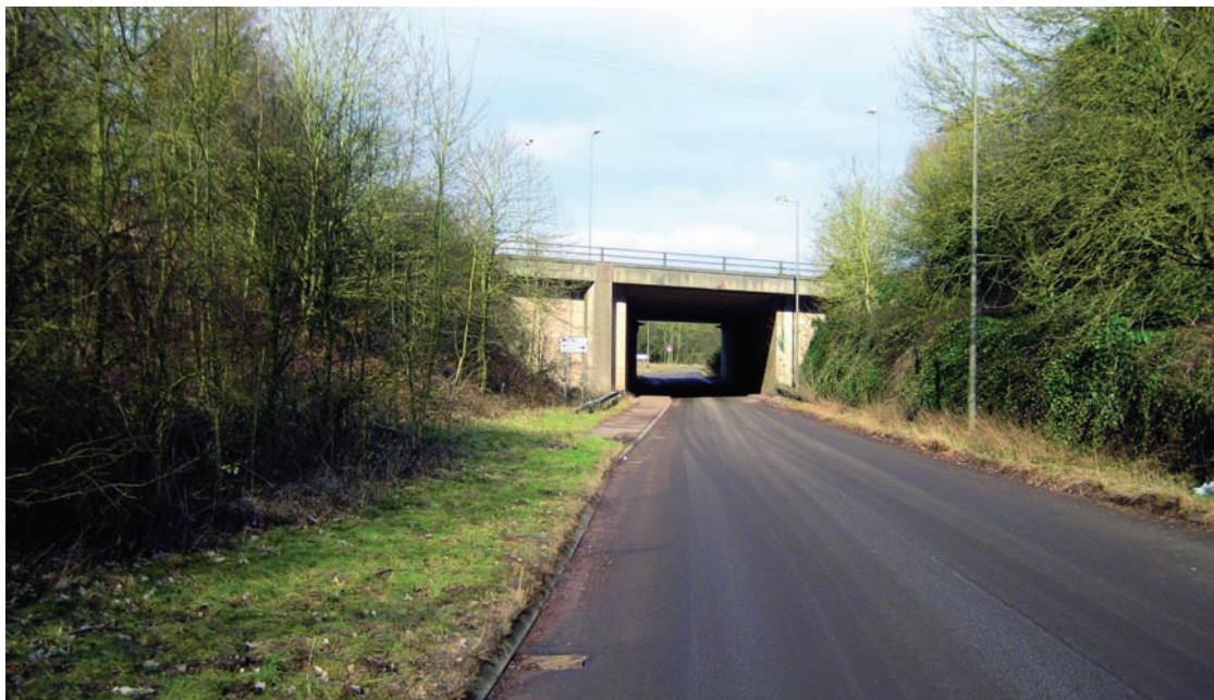
Fig 17 – This original link road to the NEC was provided beneath the A45 (before the M42 was built) along the trackbed of the original Stonebridge Railway
