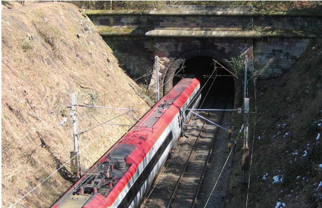
Fig 8 – The Coventry Corridor's capacity is constrained by having only two tracks, seen here passing through Beechwood Tunnel
