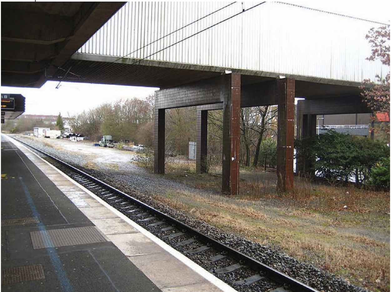
Space at Birmingham International station for an additional island platform
