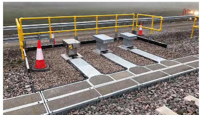
Photo 1: this is an example of a bespoke walkway kit designed and kitted off-site for delivery into EWR. In this instance it's walkway and troughing connecting into a loc base
