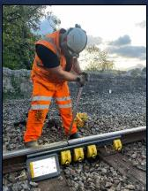
Intelligent Temporary Clamps upload telemetry to the cloud every 15 minutes providing 1344 data points logged per week.
